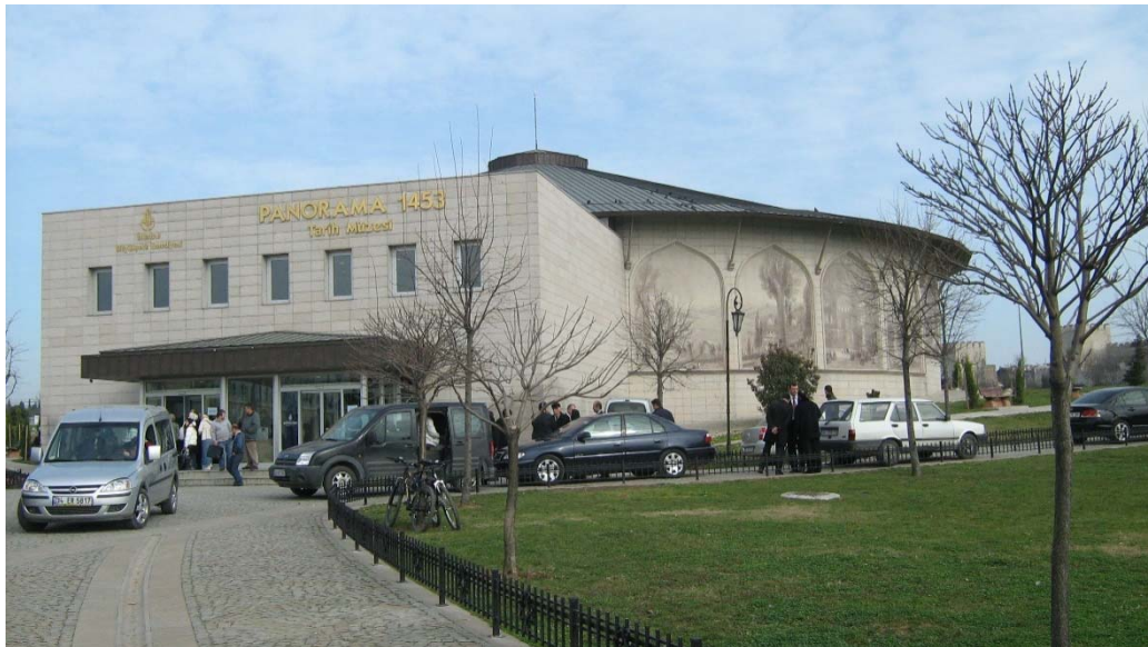
Figure 2: Exterior of the museum. Notice the circular building and the dome surrounding it (Source: İlhami DİNÇ; https://commons.wikimedia.org/wiki/File:Panorama_1453_History_Museum.JPG ), "Panorama 1453 History Museum", marked as public domain, more details on Wikimedia Commons: https://commons.wikimedia.org/wiki/Template:PD-user )
